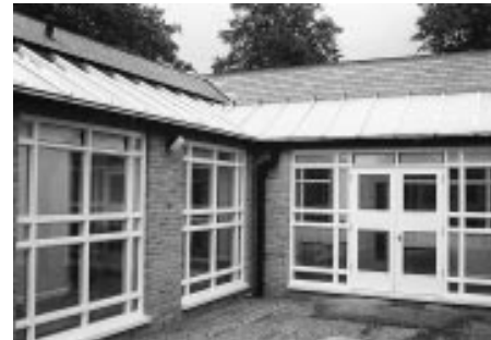
The newly completed Children's Centre due to be equipped and opened in September.
